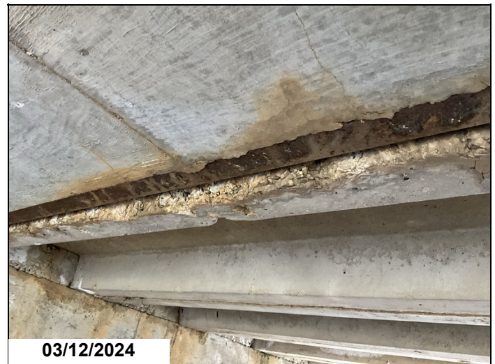
Span # 1, unit # 4, right stem-Spalling
