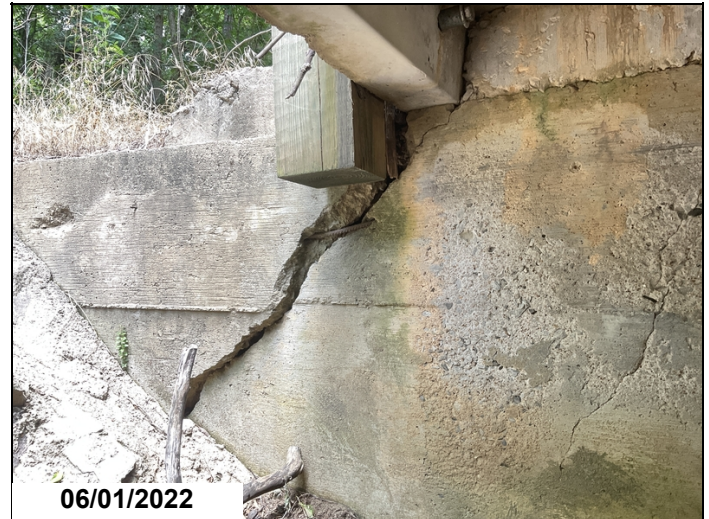
Abutment # 1, right side-Fractured under right stem of unit # 6.
