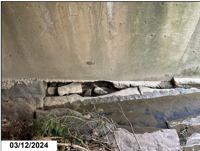
Bent 3, has irregular void under the footing. 1LF
