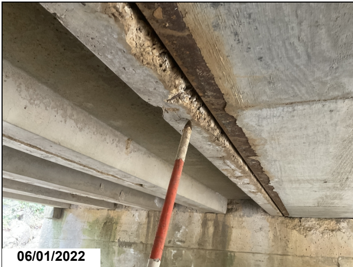
Span # 1, unit # 4, right stem-Spalling
