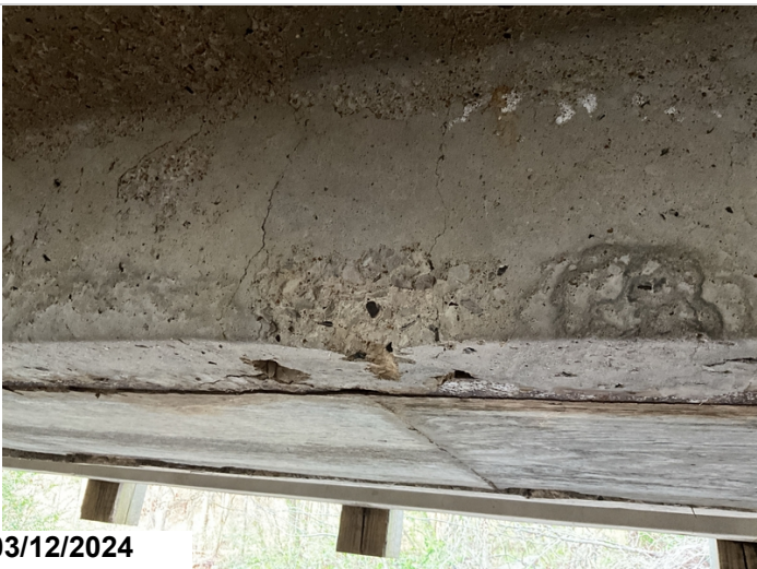
Span 1, unit 4, right leg has spalling. CS3 1LF
