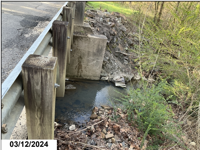
Loosely bolted rail on right side of bridge.
