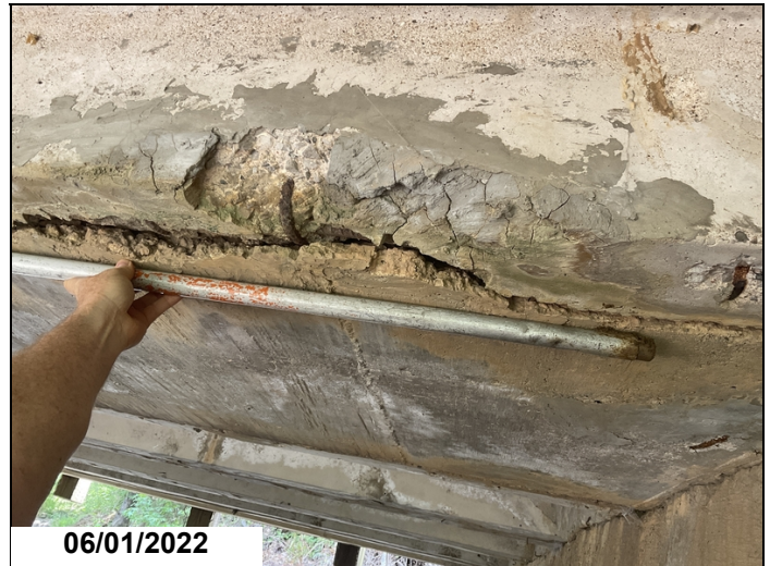
Span # 2, unit # 6, left stem near abutment 2-Failing grout repair.
