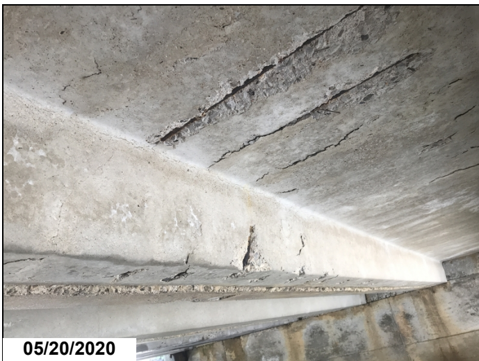
Span # 1. Channel Unit # 2. Spalls with exposed reinforcing steel.
