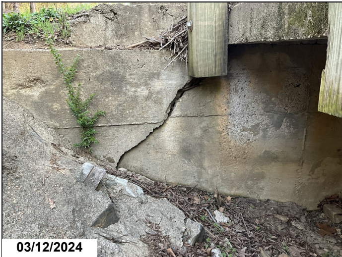
Abutment 1 on the right side has large crack. CS3
