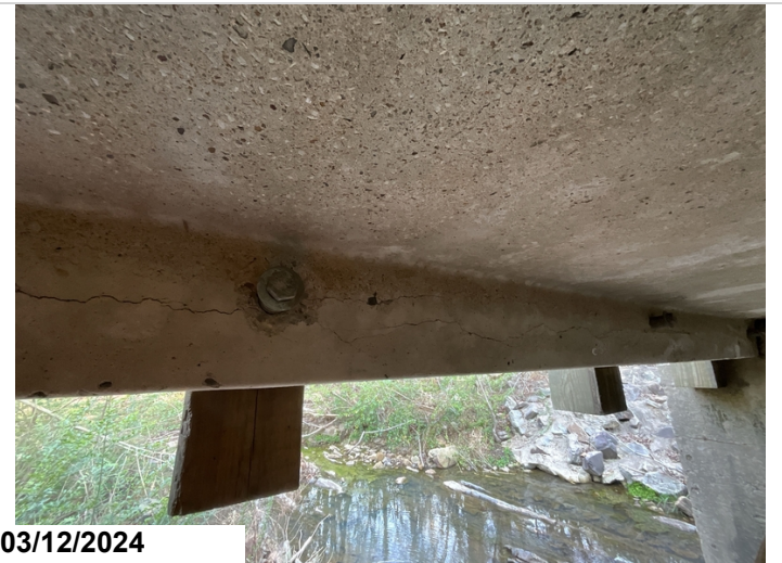
Span 2, unit 5, right leg, has cracking along the bolted guard rail. CS3 15 LF.
