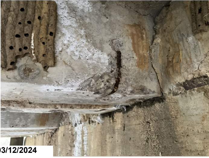
Span 2, unit 3, right leg, has spalling with exposed reinforcing steel. CS3
