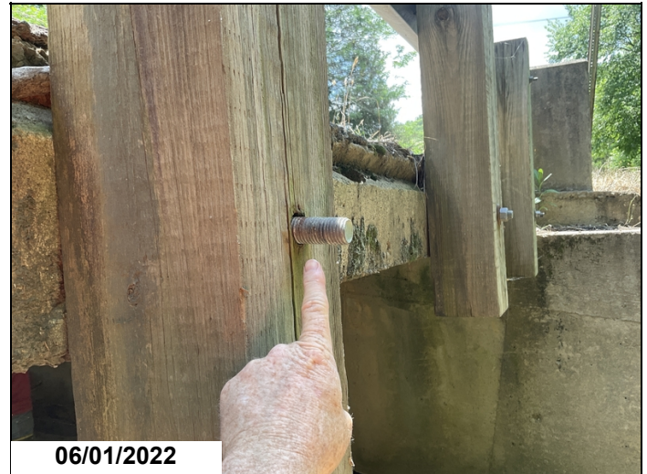
Span # 2, post # 3, right side-Missing nut on bolt that secures post to channel beam
