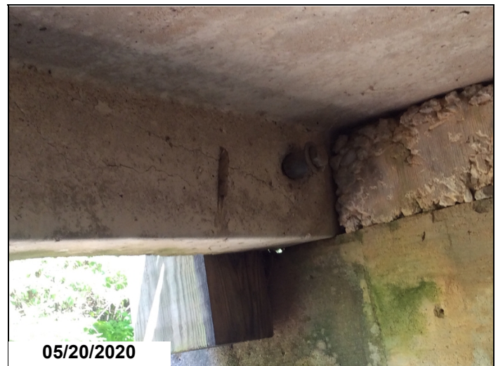
Span # 2 Unit # 6 shear type crack in the RT stem.
