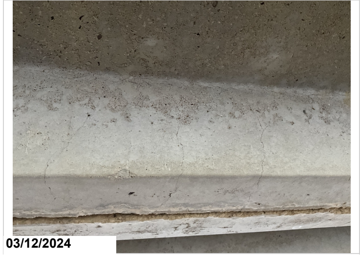
Typical flexure cracks in all units. CS2
