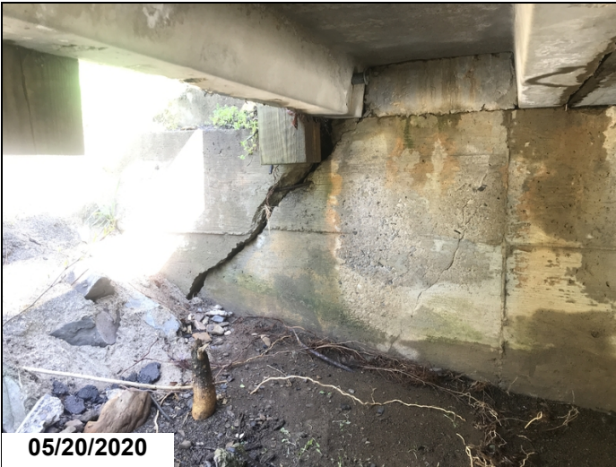
The right side of abutment # 1 stem wall is fractured and has exposed reinforcing steel. The fractured portion of the stem wall extends under the right stem of unit # 6 on the exterior side of the structure.
