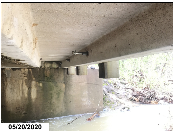
The bridge rail on the right side of the structure is loosely bolted to the exterior stem of channel units.
