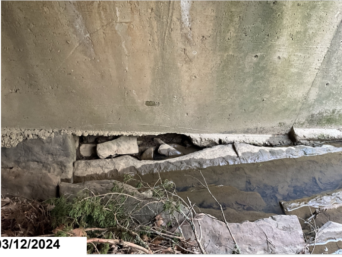
Bent 3, has irregular void under the footing. CS2 1LF
