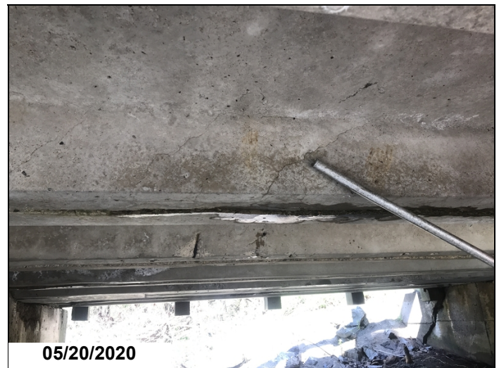
Span # 1 shear cracks in the Right stem of Channel # 1.
