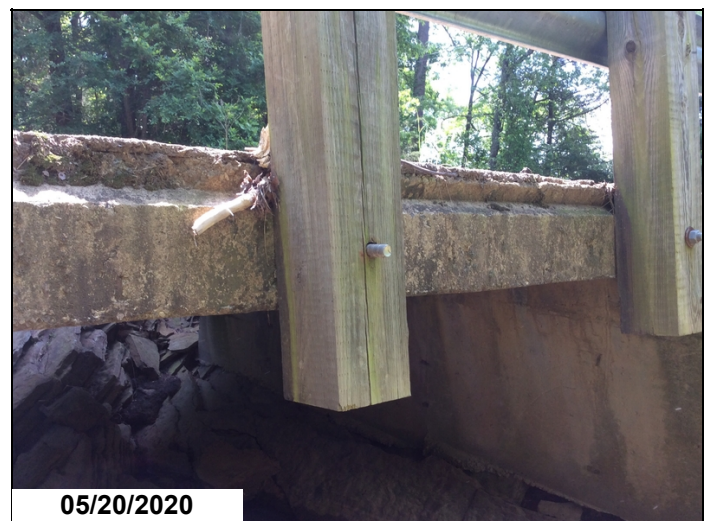
Post # 3 on the right side of span # 2 is missing a nut on the lower anchorage bolt.
