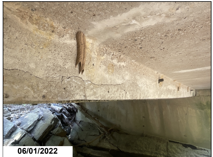
Span # 2, unit # 6, left stem has longitudinal cracking.
