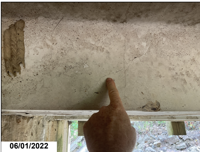
Span # 2, unit # 3, left stem-Shear type crack.
