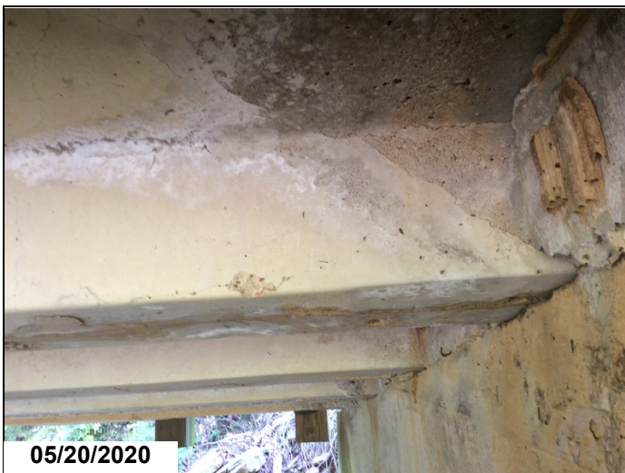
Bent # 3 Unit # 4 shear crack that extends into the deck.
