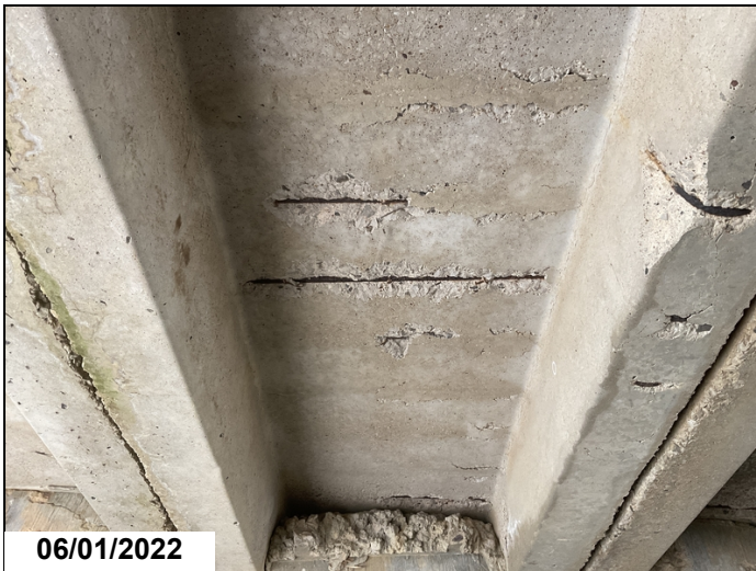
Span # 1, unit # 2-Spalling with exposed reinforcing steel in deck undersurface.
