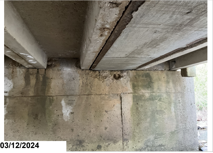
Pier 2, back side in the bearing area has large spall. CS3 2LF
