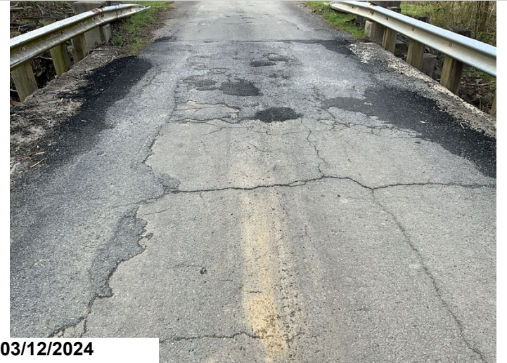
Vertical and horizontal cracking in the overlay full length of deck. CS3 Cracking
