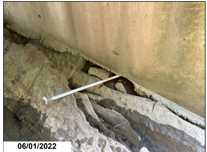
Abutment # 2 has a 3' long x 5" tall void that penetrates up to 16" under the base of the abutment that is located under Unit # 5. Bent appears to be constructed on non-uniform solid rock channel with no apparent scour problems during this inspection.
